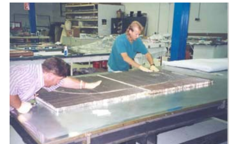
Painel BDR/Shunt com HPs imbutidos
